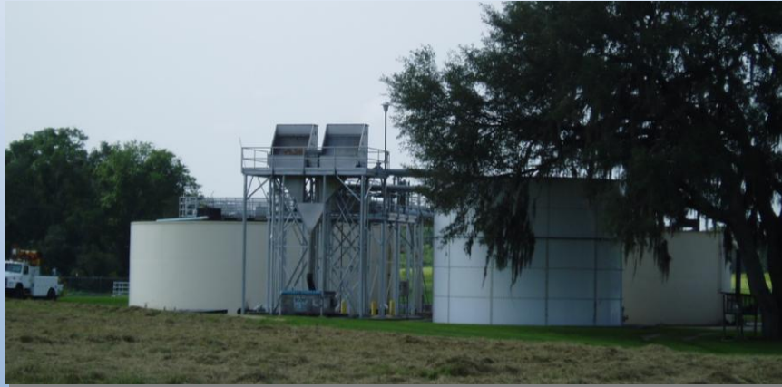
The headworks, carousal, and equalization basin at the City of Newberry WWTF
