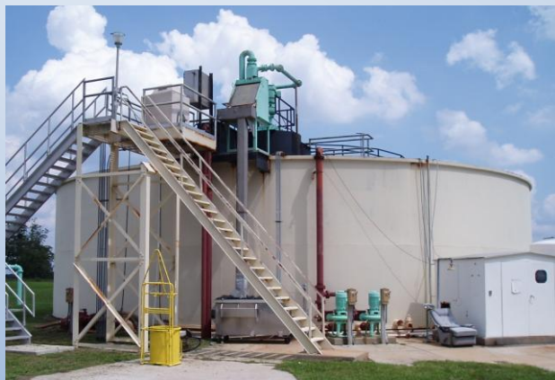
The City of Hawthorne Wastewater Treatment Facility
