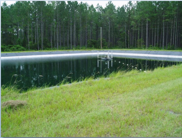
An aeration basin at the Gainesville Raceway WWTF
