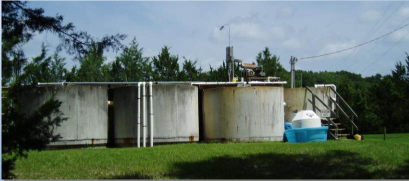
Aeration basins, clarifier, and chlorine contact chamber at the Camp Kulaqua WWTF.
