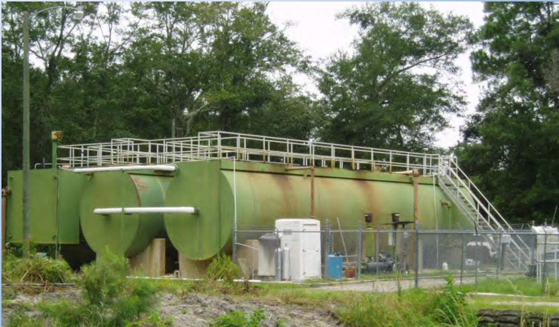
The aeration basins, digester, and clarifier at the Waldo WWTF
