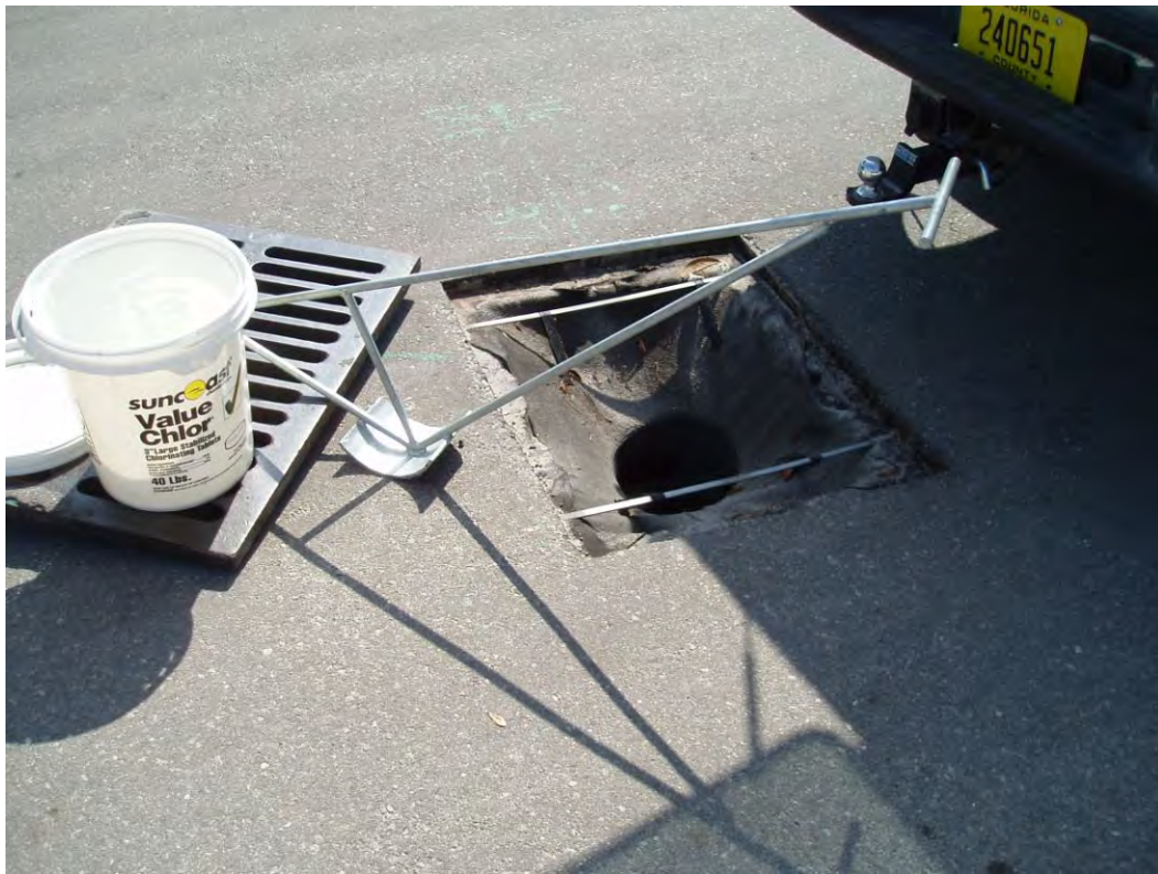
Removal of stormwater inlet grate
