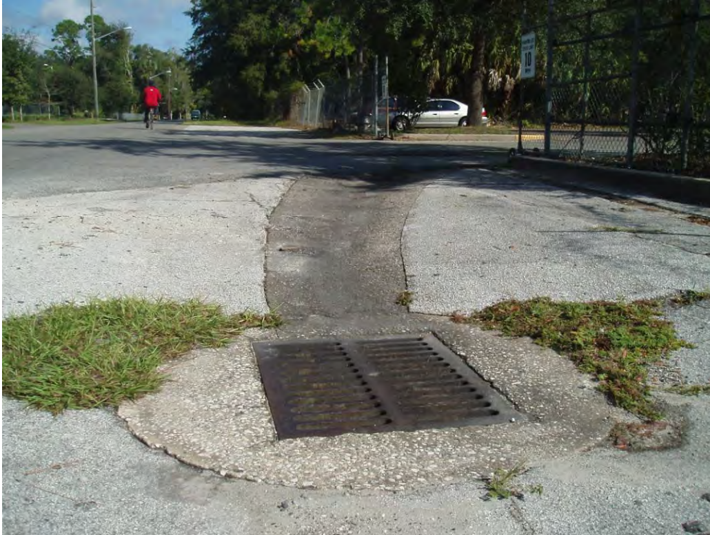
Florida Pest Control & Chemical Company North Inlet next to NW 2 nd Street
