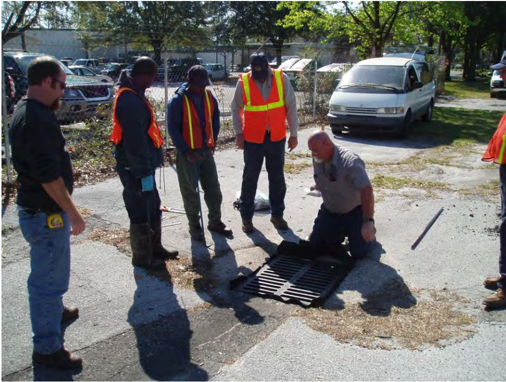
Installation of inlet filter and trimming excess filter material
