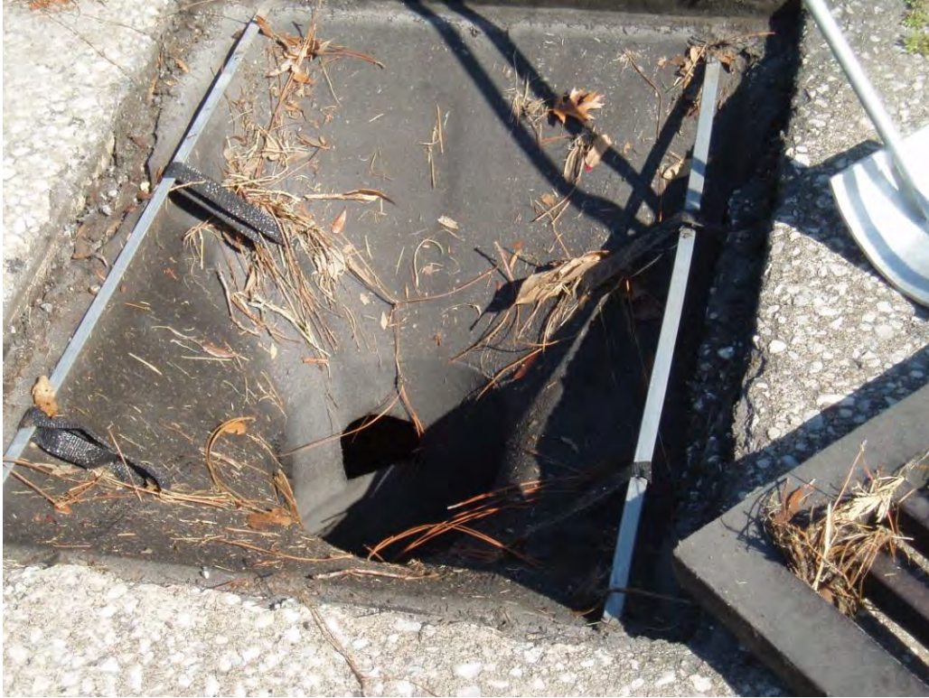
Inlet filter in place and attached to tension bars, immediately prior to removal
