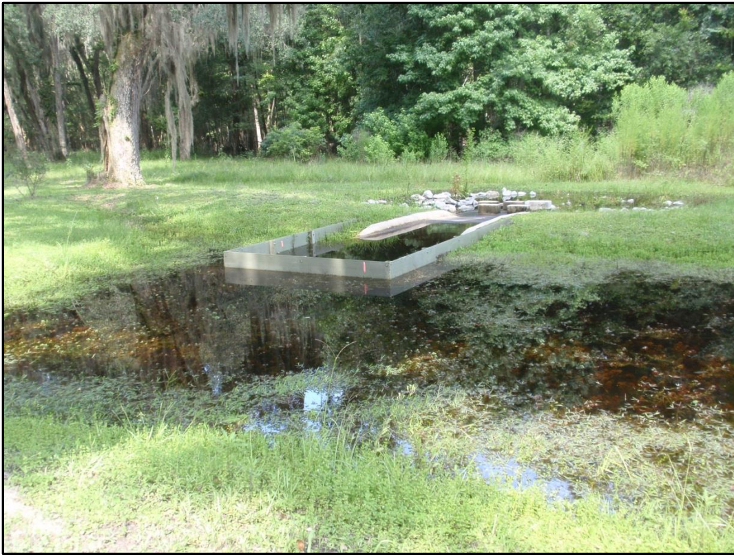
Owens-Illinois Stormwater Pond (July 26, 2013)
