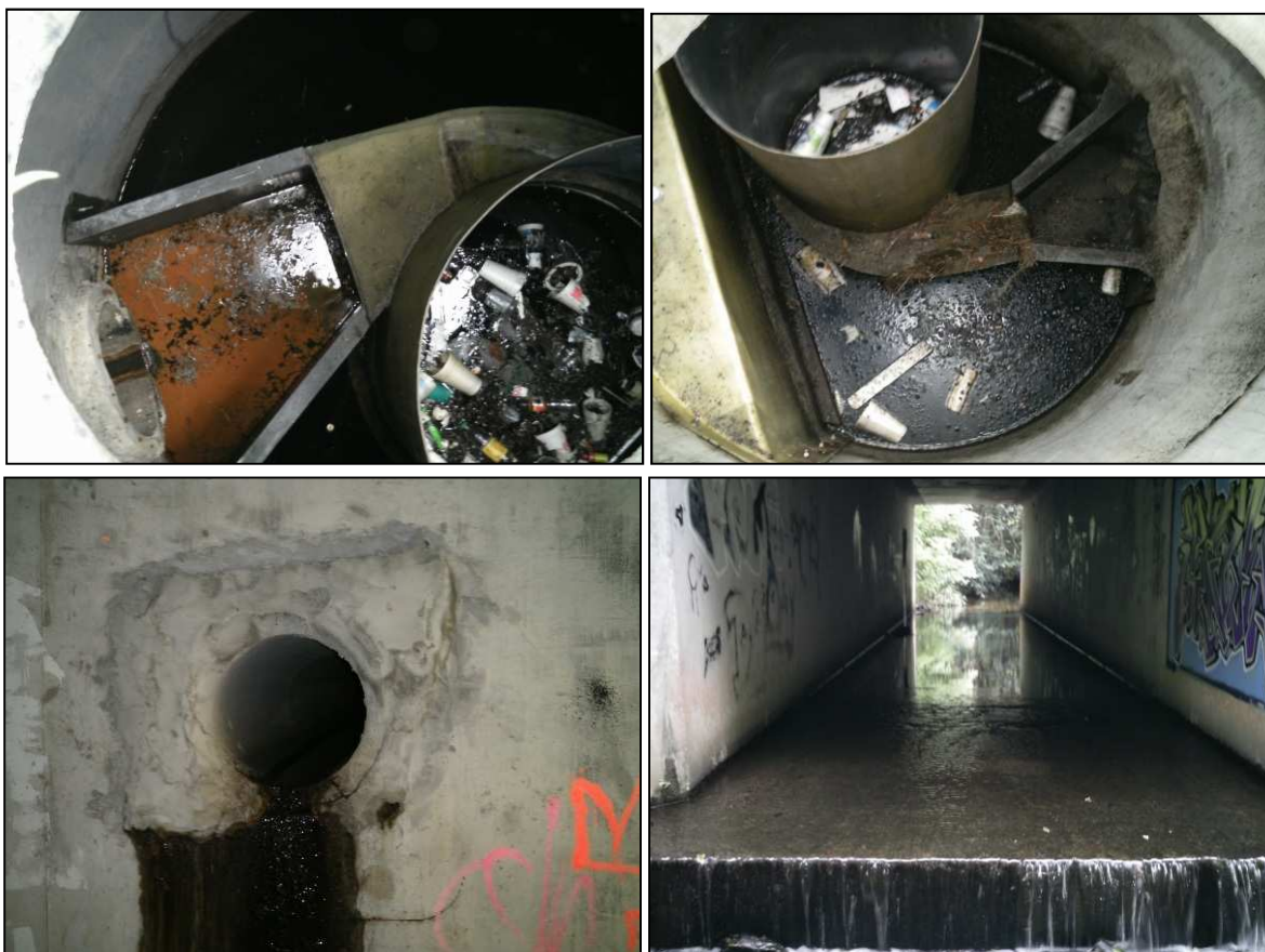
Figure A-1. From top left to bottom right, HOG29-W Vortex and Main Chambers, HOG29-E Vortex and Main Chambers, the HOG29-W outfall pipe, and the HOG29DS downstream sample location. June 19, 2012
