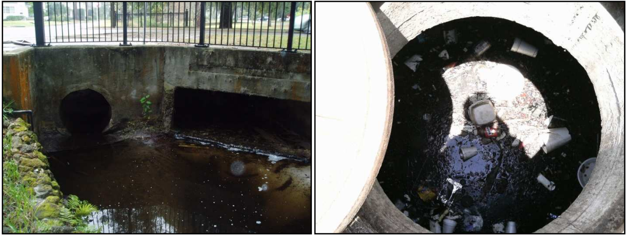
Figure A-3. Outfall pipe from SWB8 and Sweetwater Branch culvert (left) and SWB8BOX (right). December 12, 2012 and June 19, 2012
