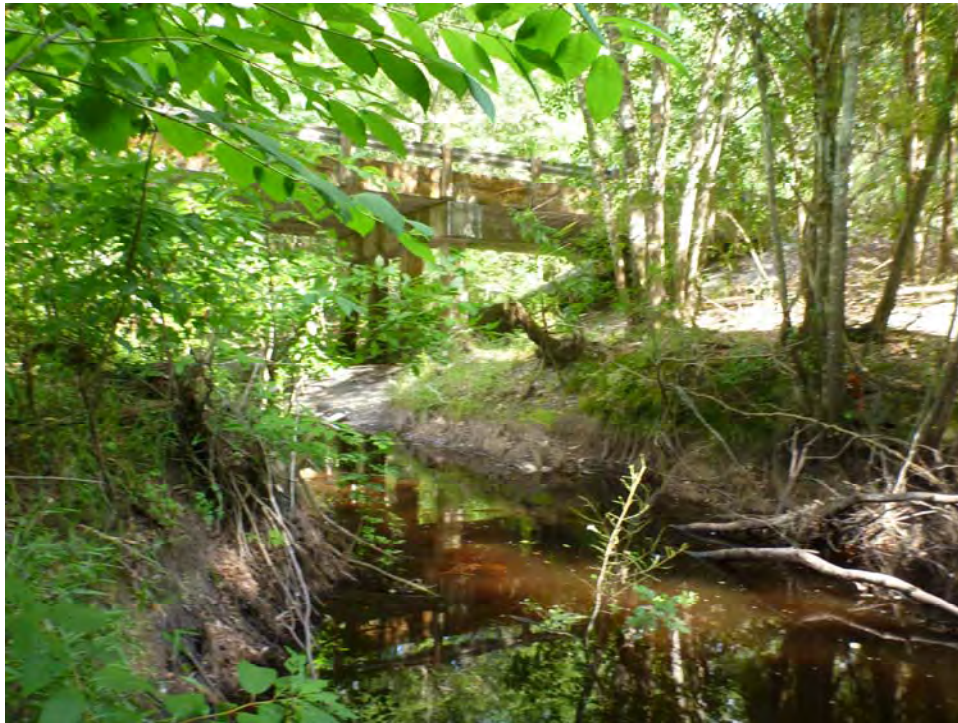
Looking upstream SFR010C1
